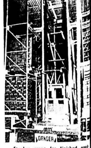
Stacker crane for finished goods.
